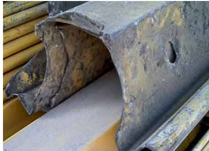
Toeboard Steel UPY ■ flange of toeboard is bent
