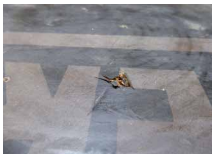
Nail holes (nailed at the rear)
