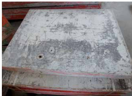
Non-removable dirt ■ Sheet replaced
