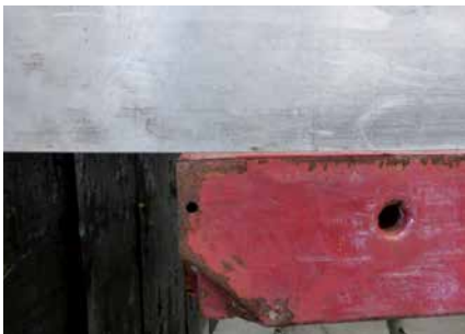
Element bent > 8 mm
