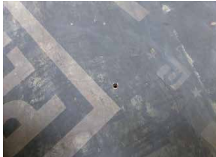
Nail holes (nailed at the front)
