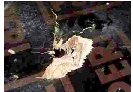
Holes >math>\gt; \varnothing 35 \text{ mm}</math> ■ Sheet replaced
