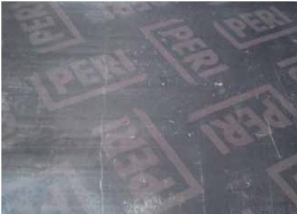
Damage \leq 1 mm deep
